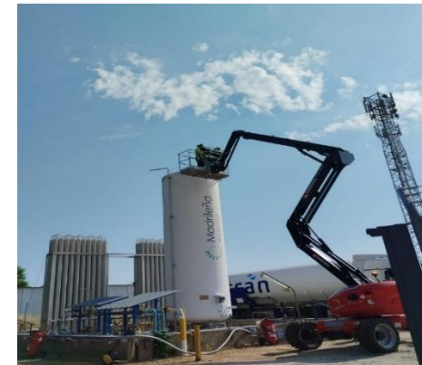
Repair work on the outer casing of the Talamanca de Jarama tank
