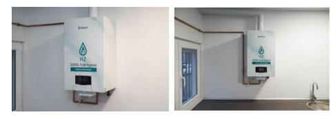
Image 42 Boiler installed at Madrileña Red de Gas offices with 100% hydrogen consumption
